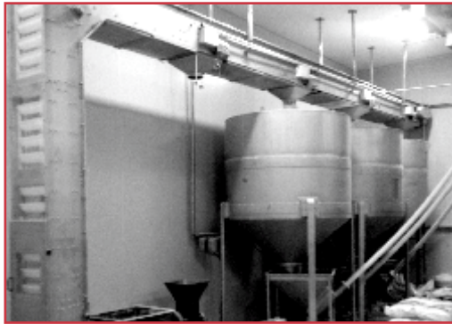
Automatic Weigh Based Conveying, Storage & Processing
